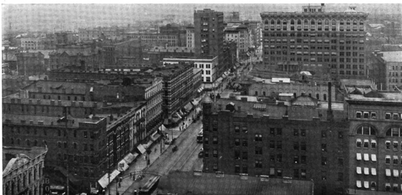
LOOKING NORTH ON HIGH STREET, COLUMBUS, SHOWING SHOPPING DISTRICT
