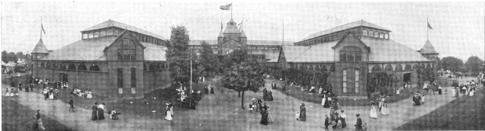
PART OF THE MAIN BUILDINGS AT THE FAIR GROUNDS, COLUMBUS
